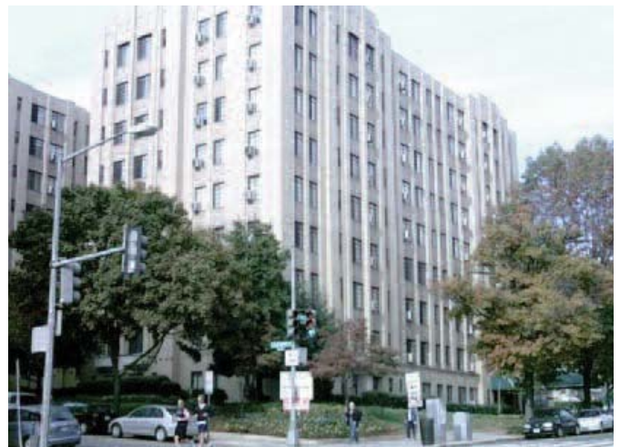
Apartment building, built in 1923, underwent a total renovation of its A/C system. Ninety five "Junior bedrooms" used AireShare transfer fans for comfort.
